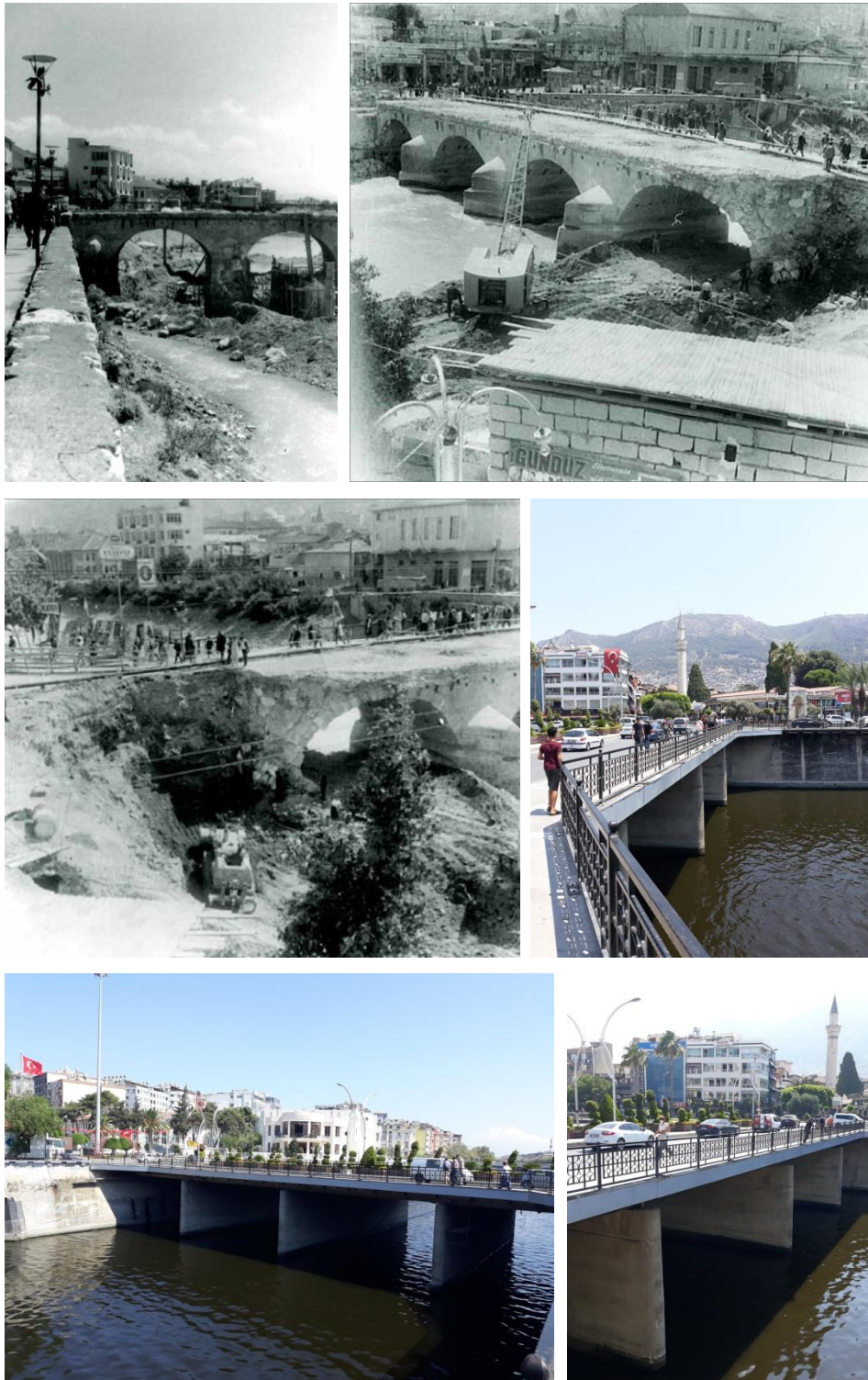
Figure 4.36. The demolition of the bridge, from 1972 (the black and white ones are from the demolition of the bridge, from 1972 and the colored ones are the new bridge later built on the same place, at present) (Ovalı, 2017, p. 151; 152; 153; taken from the authors personal archive)
