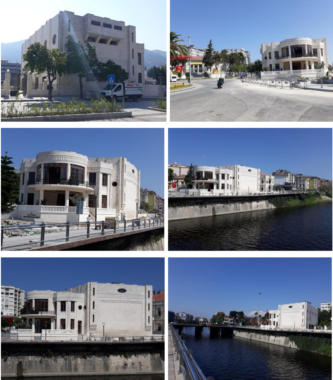
Figure D. 1. Meclis Culture and Art Center (old Gündüz Cinema and old Parliament building) (taken from the author's personal archive)
